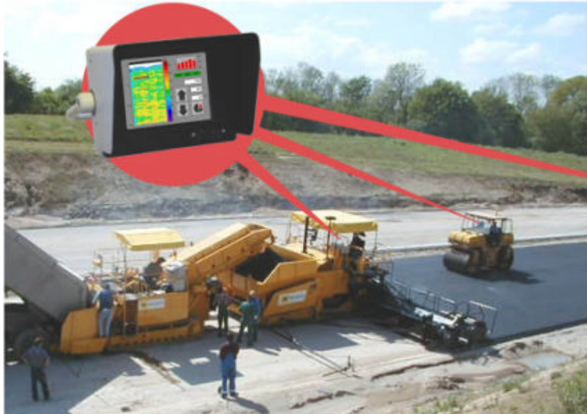
Figure 4. Continuous Asphalt Compaction on BAB A20.
